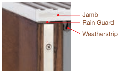
Top of door; exterior view.
